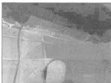
Photo N° 1922 AMIANTE CIMENT -Rdc-Chaufferie Clapets Plaques planes (Fibres-ciment)
