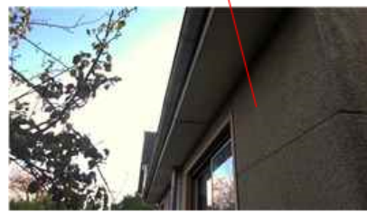
Façade Nord Plaques amiante ciment
