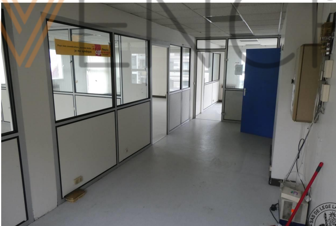
46 Couloir de distribution
